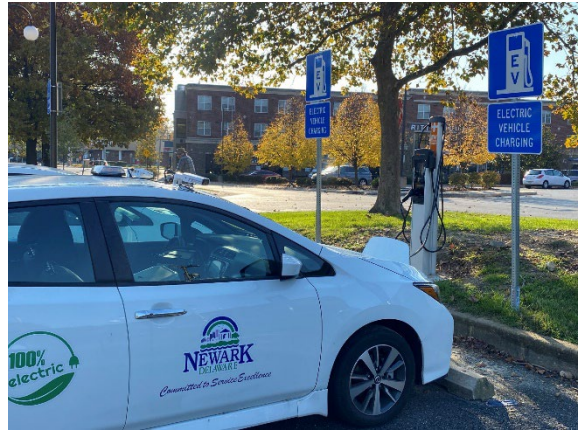
AN ELECTRIC FLEET VEHICLE FOR THE CITY OF NEWARK CHARGES AT CITY HALL USING A CHARGING STATION MADE POSSIBLE BY DELAWARE'S ELECTRIC VEHICLE CHARGING EQUIPMENT REBATE PROGRAM
