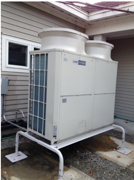
Police Station central heat pump installed as part of HVAC project
